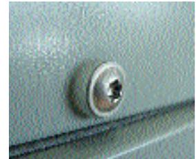
*Stainless steel screw with plastic seal*
